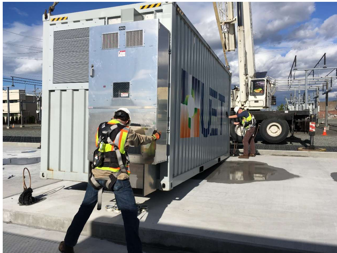
PCS Container Installation
